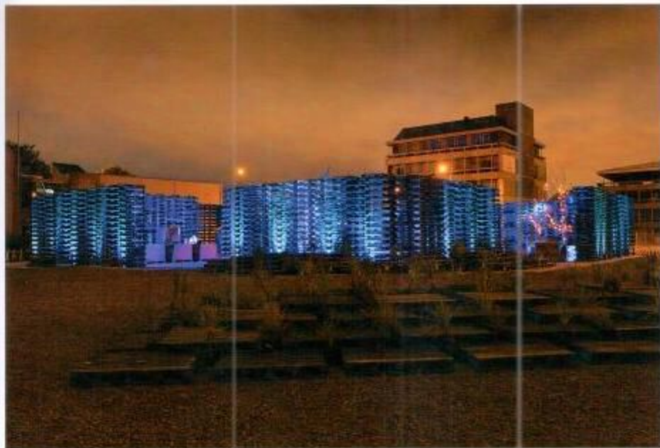
AS THE PALLET PAVILION WAS CONSTRUCTED FROM 3000 BLUE WOODEN PALLETS. PHOTOGRAPHY: MURRAY JEWIS.
